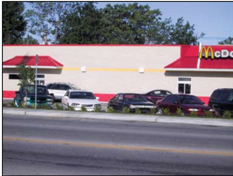
Figure 1: Exterior View of a CMU Wall Taken with a Digital Camera
